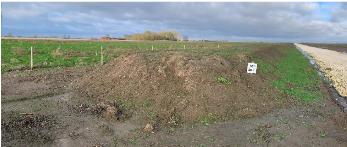
Insert 8: Temporary Topsoil Storage (January 2023)
