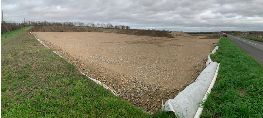
Insert 2: Example temporary construction compounds
