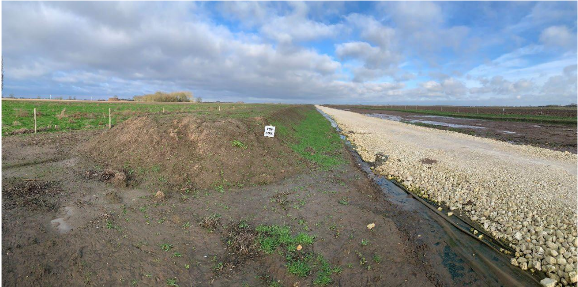
Insert 13: Temporary Topsoil Storage (January 2023)
