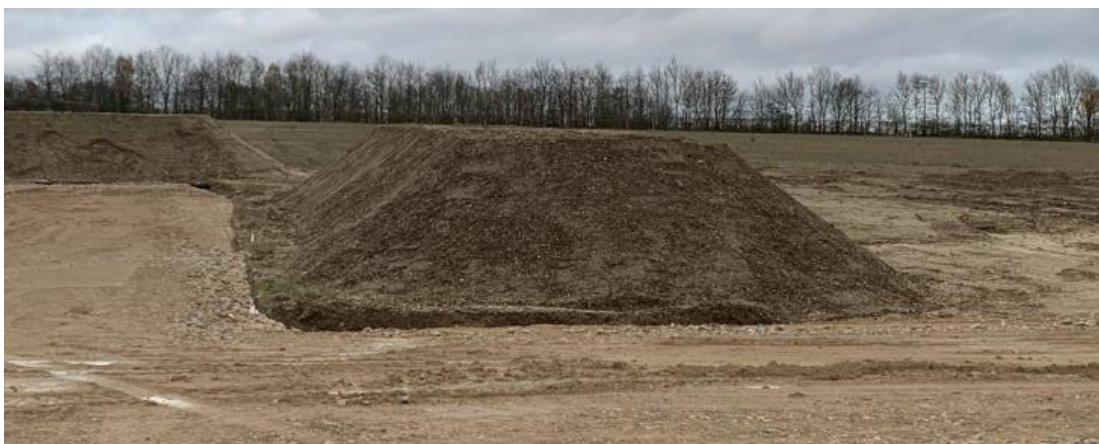
Insert 9: Construction compound for the Elsham – Lincoln water pipeline
