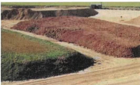
Clearly defined stockpiling of different soil materials
