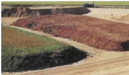
Clearly defined stockpiling of different soil materials
